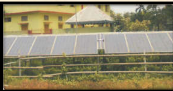
50 KWp solar power generator
