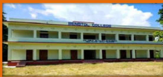
RUSA Funded New Class Rooms
