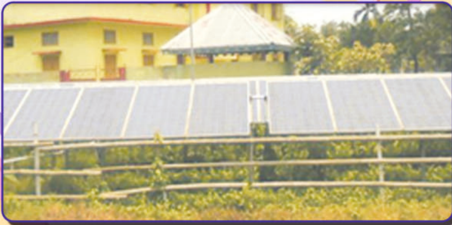
50 KWp Solar Power Generator
