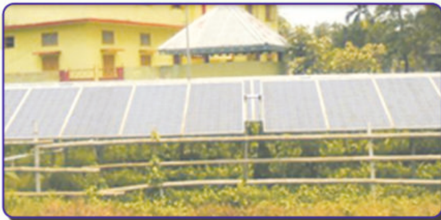
50 KWp Solar Power Generator
